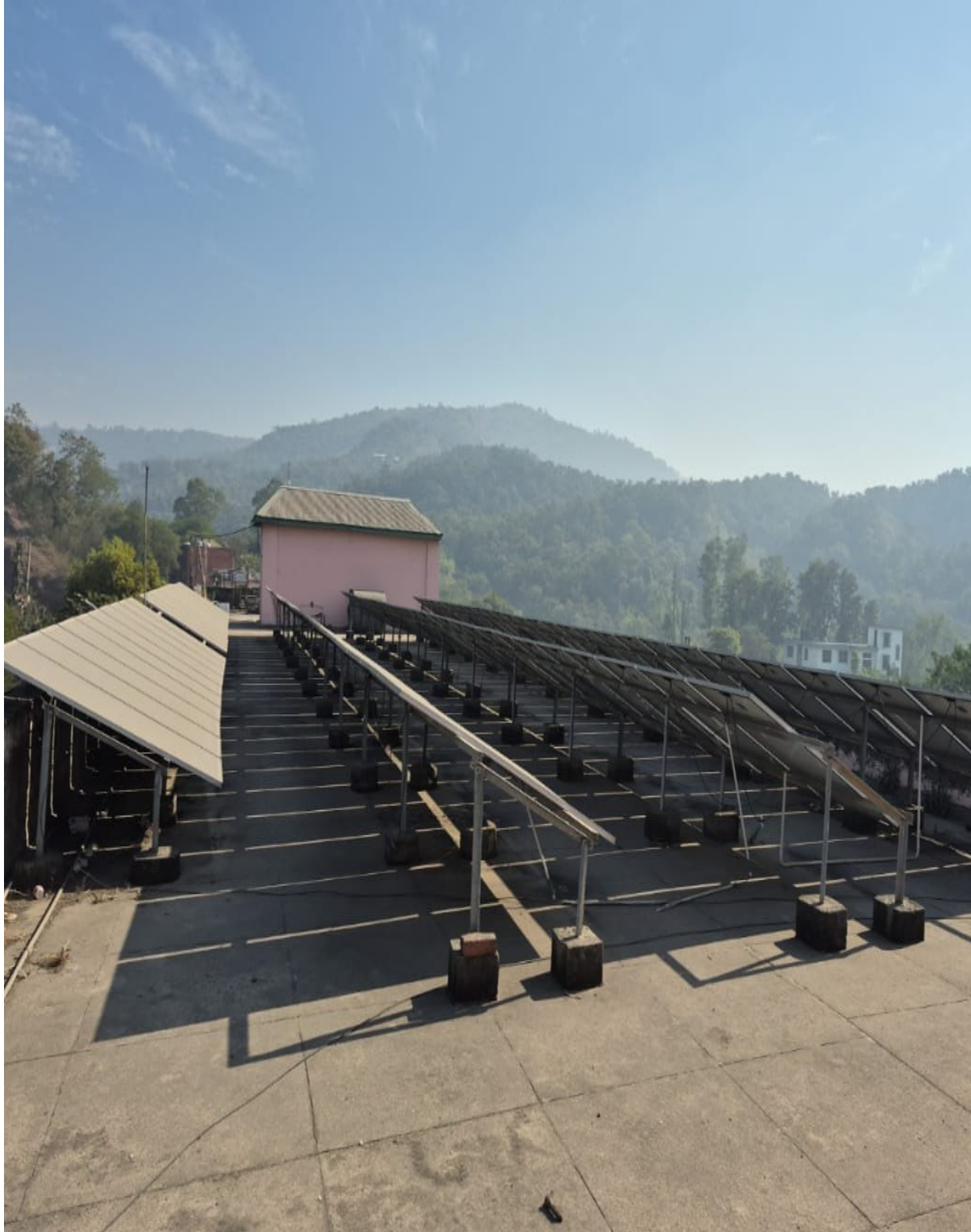
Roof-top Solar Grid: A 35 KW solar grid with a two-way meter system
